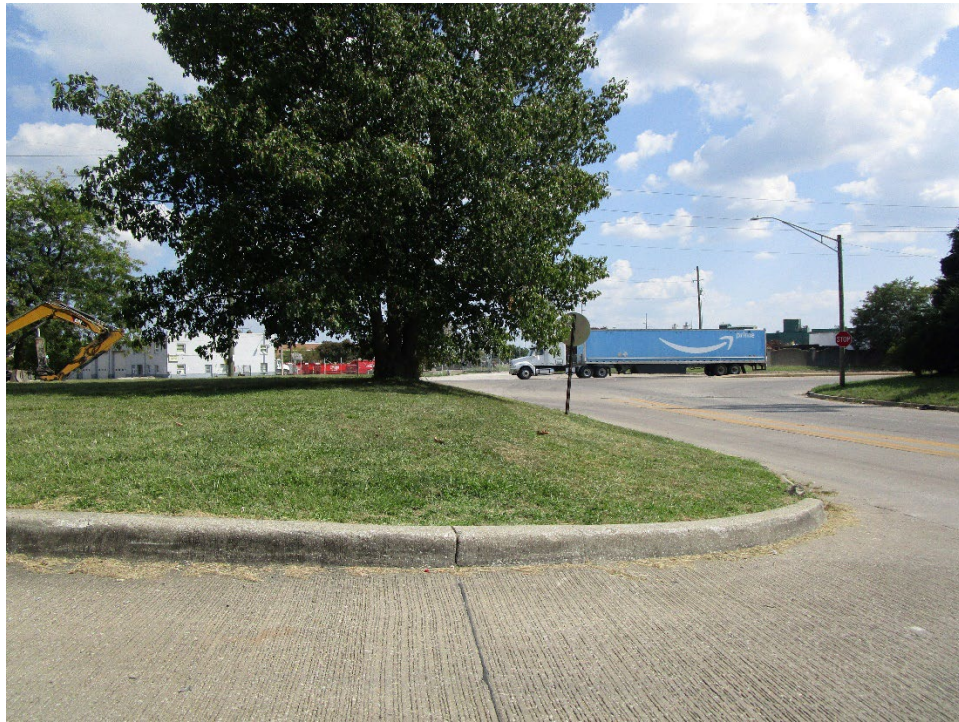
View of site looking east across Minnesota Way
