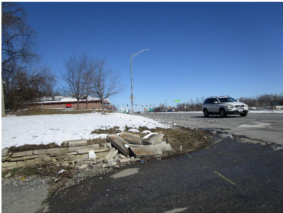
View looking north along Kentucky Avenue
