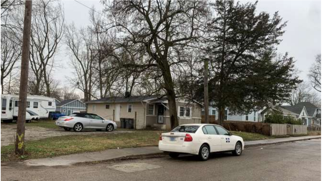
Photo of single-family dwellings west of the site.
