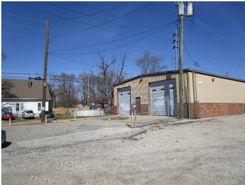
View from site looking northeast
