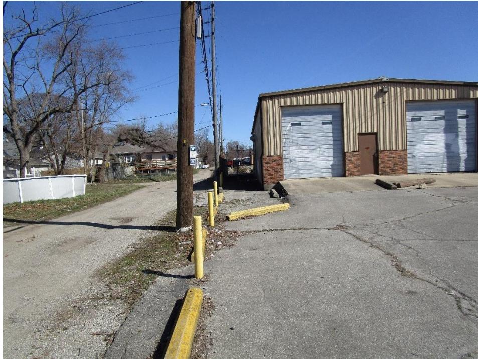
View looking east along the east / west alley
