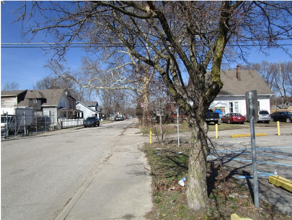
View looking north along North Bradley Avenue
