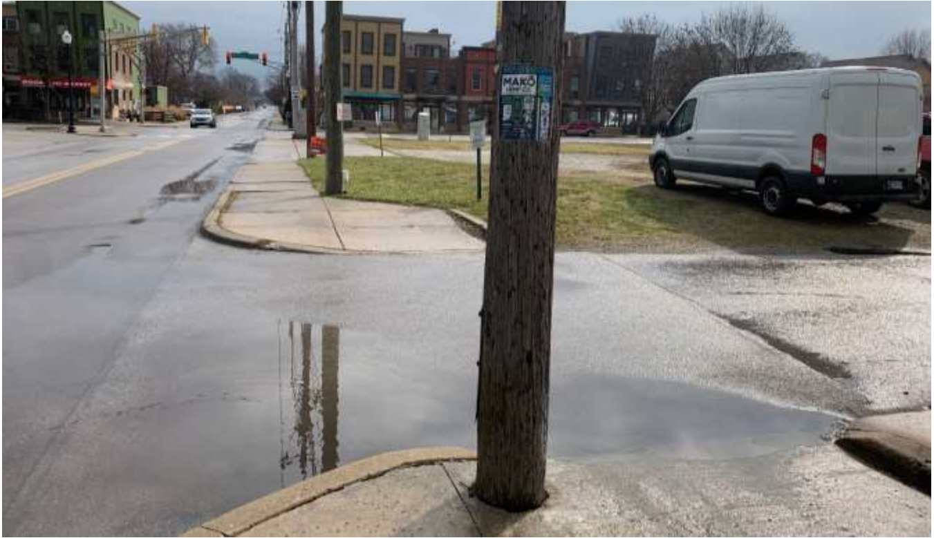
Photo of the street frontage along 25 th Street at 2460 North Delaware Street.
