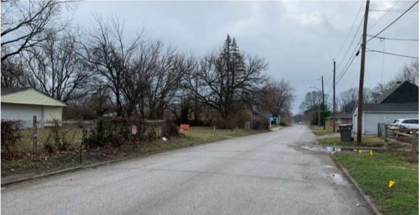
Photo of the subject site street frontage looking south on Barnes Avenue.
