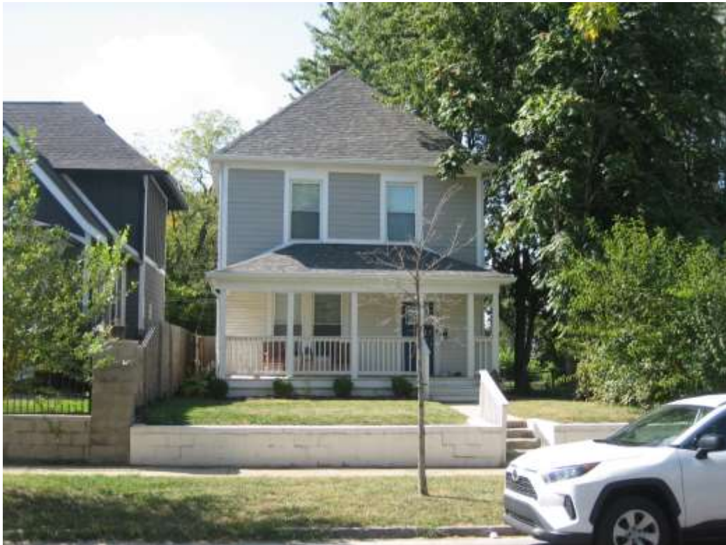
Single-family dwelling to the west of the site.
