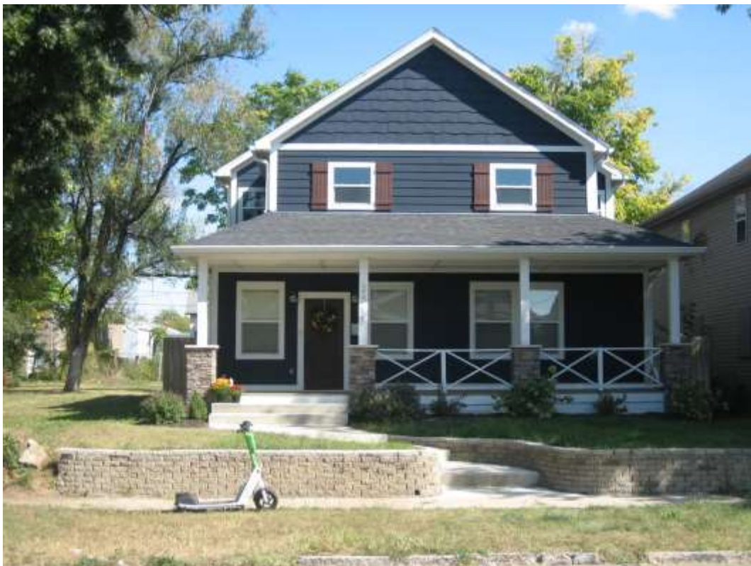
Single-Family Dwelling to the south of the site, looking east.
