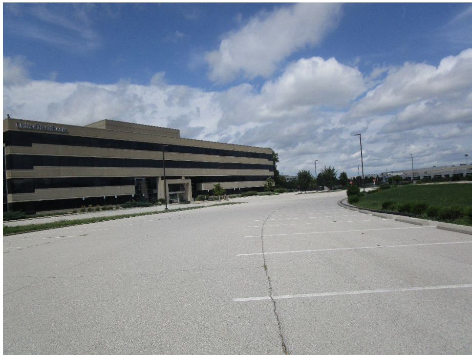
View of site looking north
