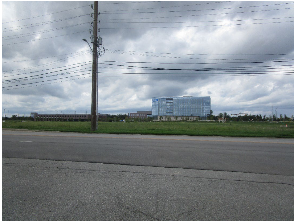
View from site looking north across Oliver Street
