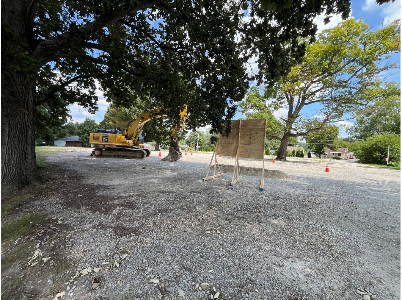
Photo 5: View of subject site from the west
