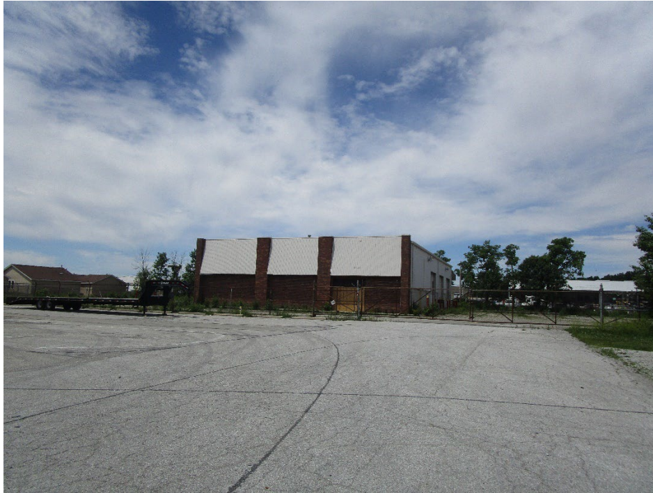
View of rear on-site building looking north
