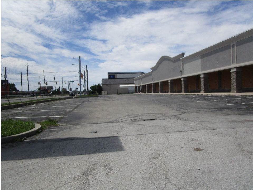
View of site looking west along West 86 th Street
