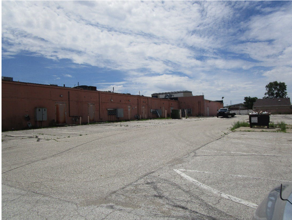
View of rear of site looking southwest
