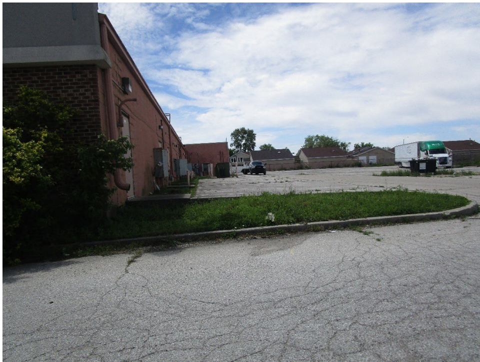
View or rear of site looking west across access drive
