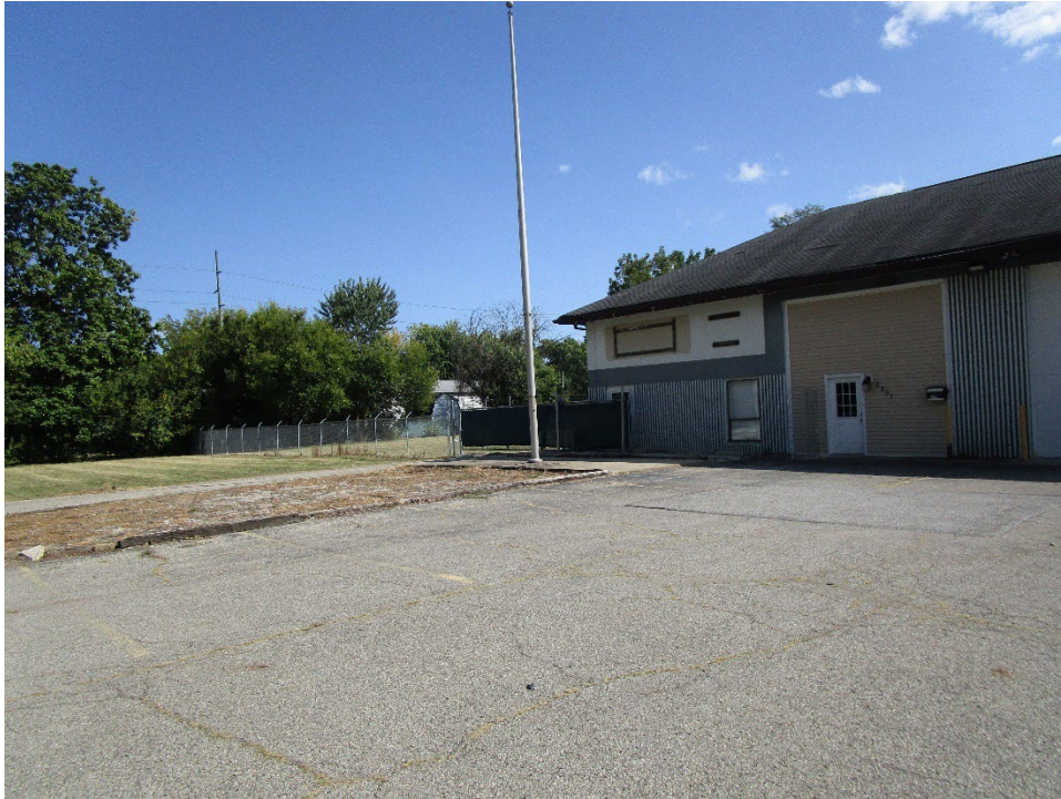
View of site looking southeast
