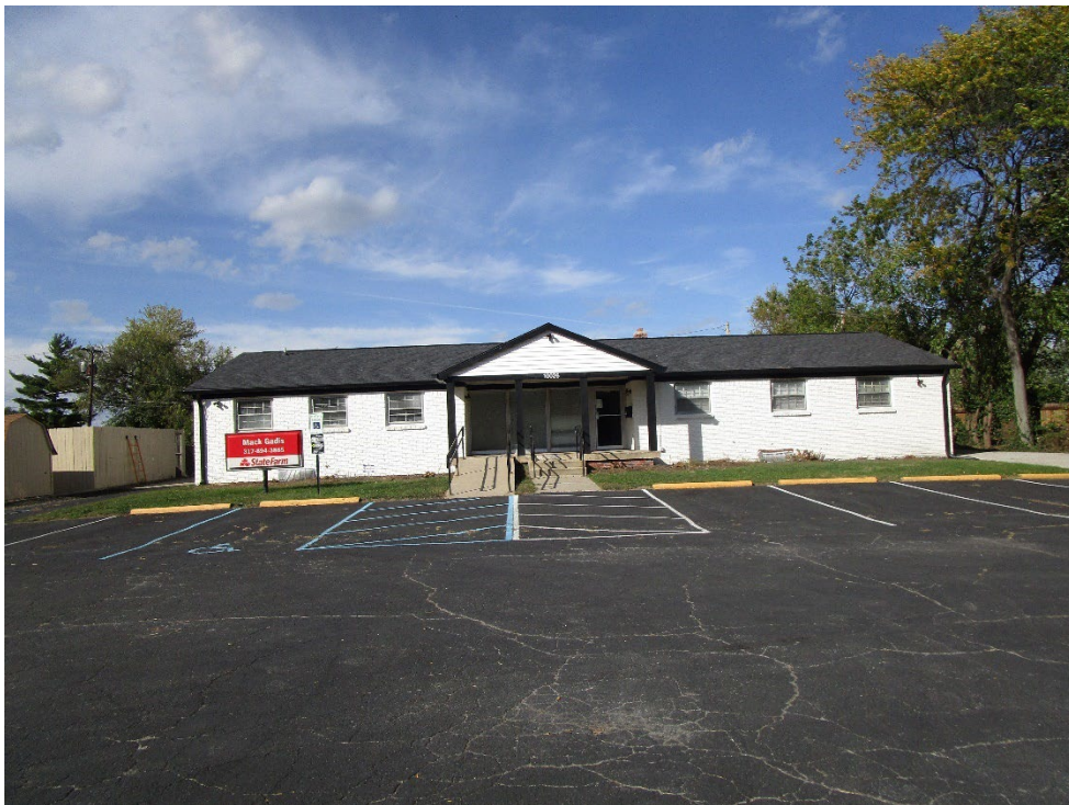
View of site looking north
