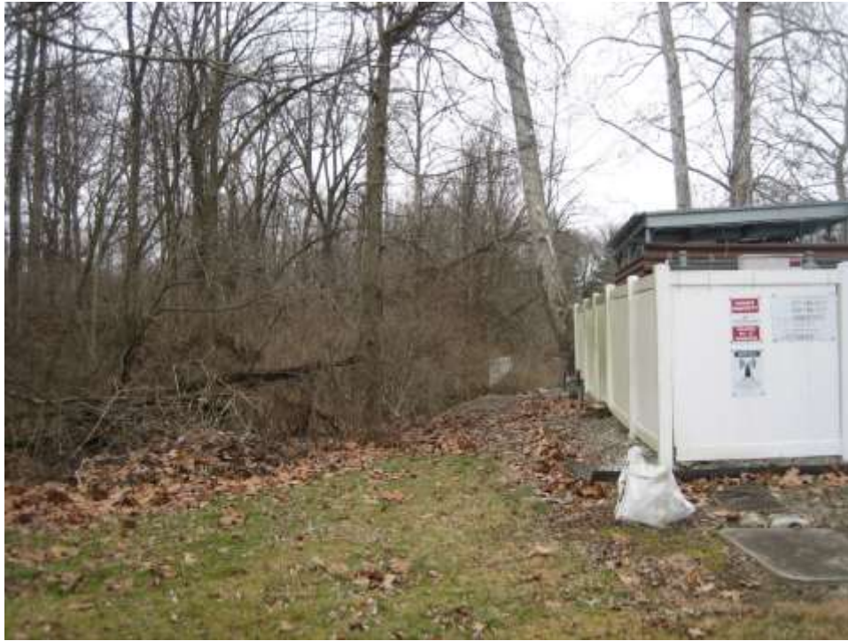
Existing wireless communication facility with seven-foot south side setback, looking west
