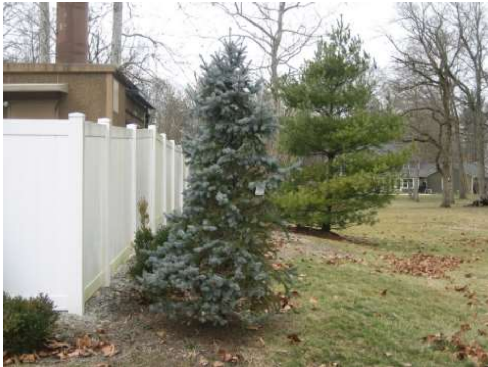
Existing wireless communication facility with 0.5-foot north side setback, looking west
