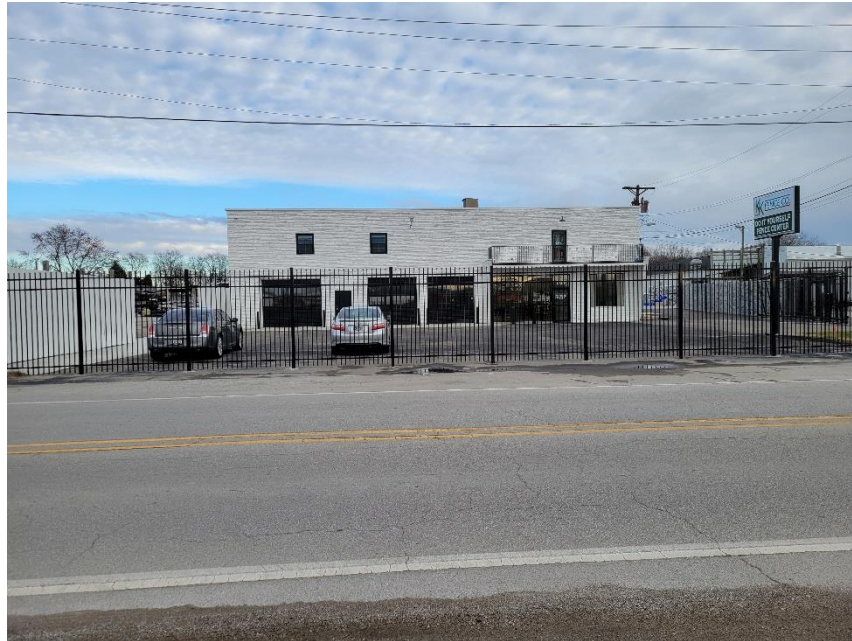
Photo 1: View of the Subject Site (from West)
