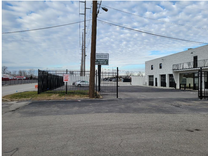
Photo 3: Fence from South
