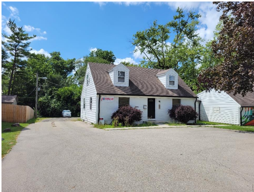
Photo 2: Offices at Subject Site
