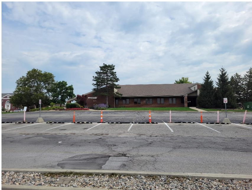
Photo 10: Adjacent Property to North
