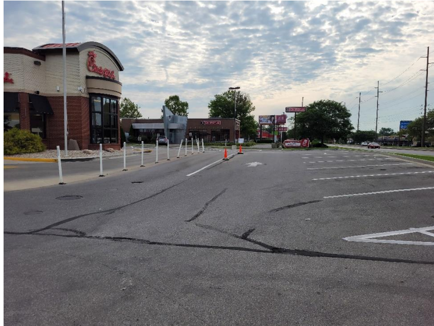
Photo 7: Southern Drive-Through Lanes Viewed from West
