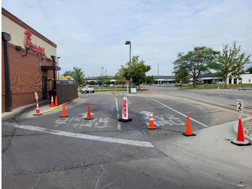
Photo 5: Drive-Through Entrance Viewed from East
