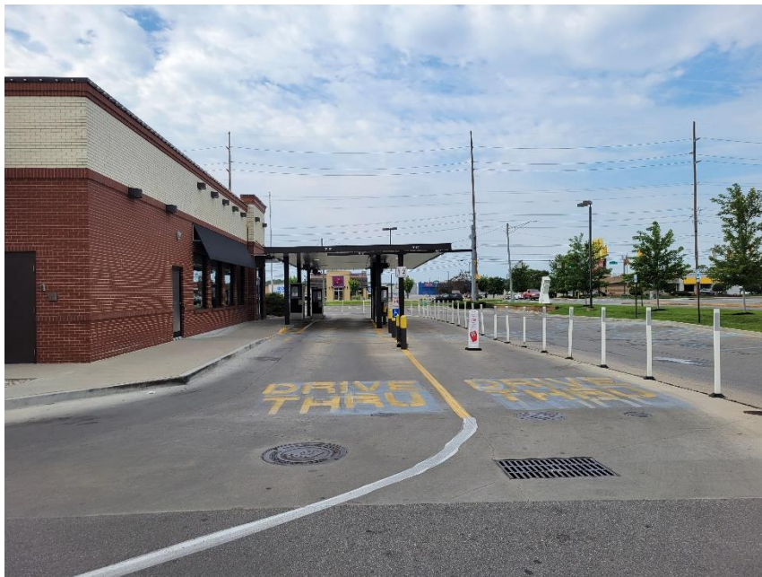
Photo 6: Existing Western Canopy + Drive-Through Lanes Viewed from North
