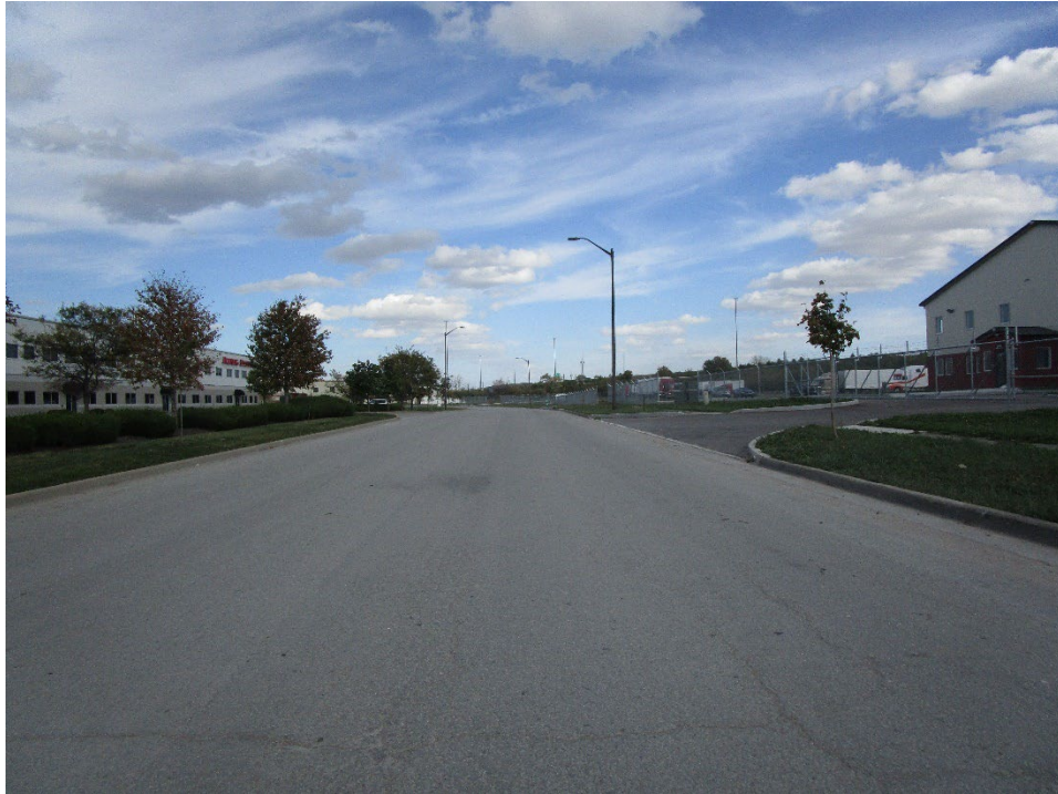
View looking east along Enterprise Park Place
