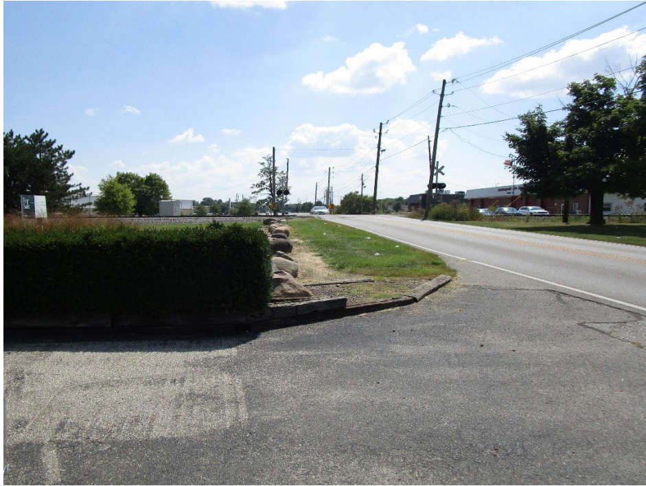
View looking south along South Franklin Road
