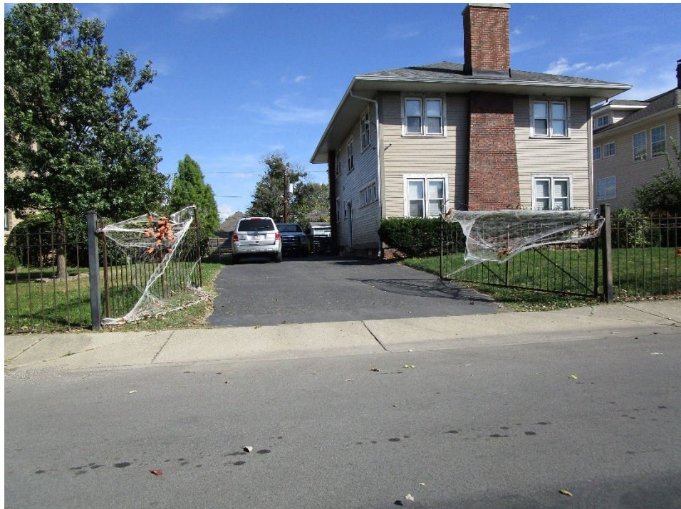
View of site looking east across Ruckle Street
