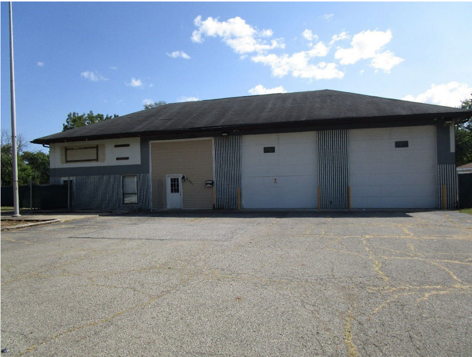
View of site looking south
