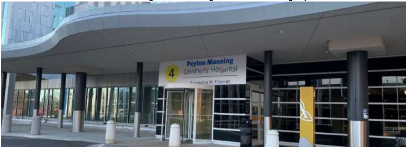
Photo of a wall sign not included in the request along the eastern building façade that would need an approval petition.
