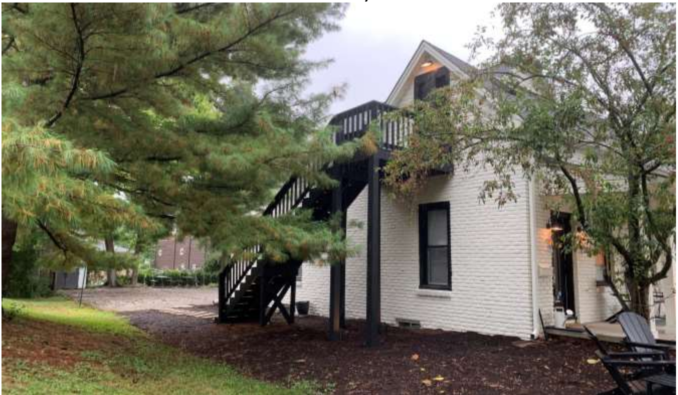
Photo of the staircase that leads to the dwelling unit on the second floor.
