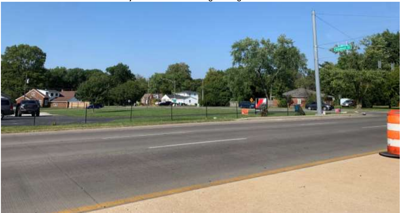
Subject site street frontage along 10 th Street.
