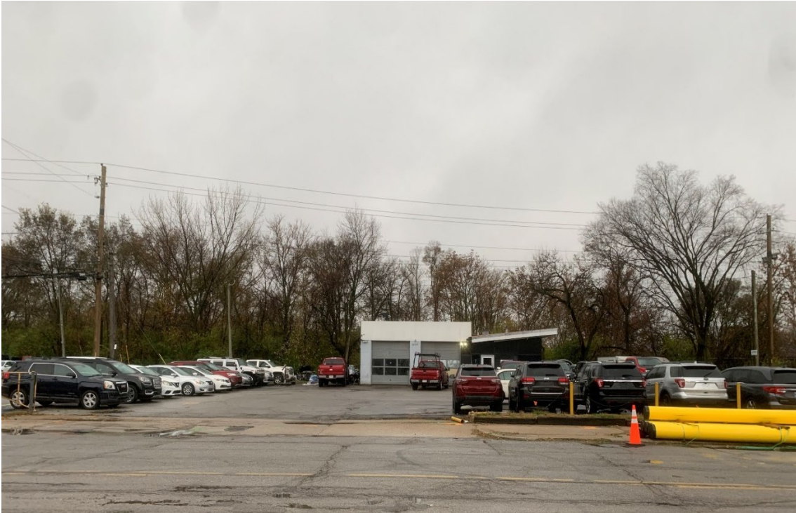
View of site looking south across West Washington Street
