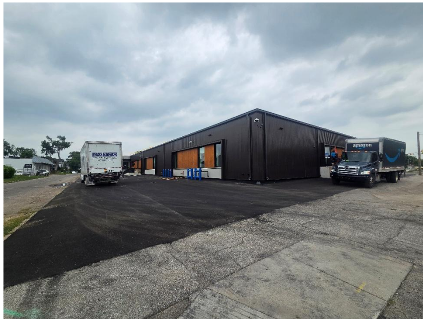
Photo 6: Building Viewed from Southwest
