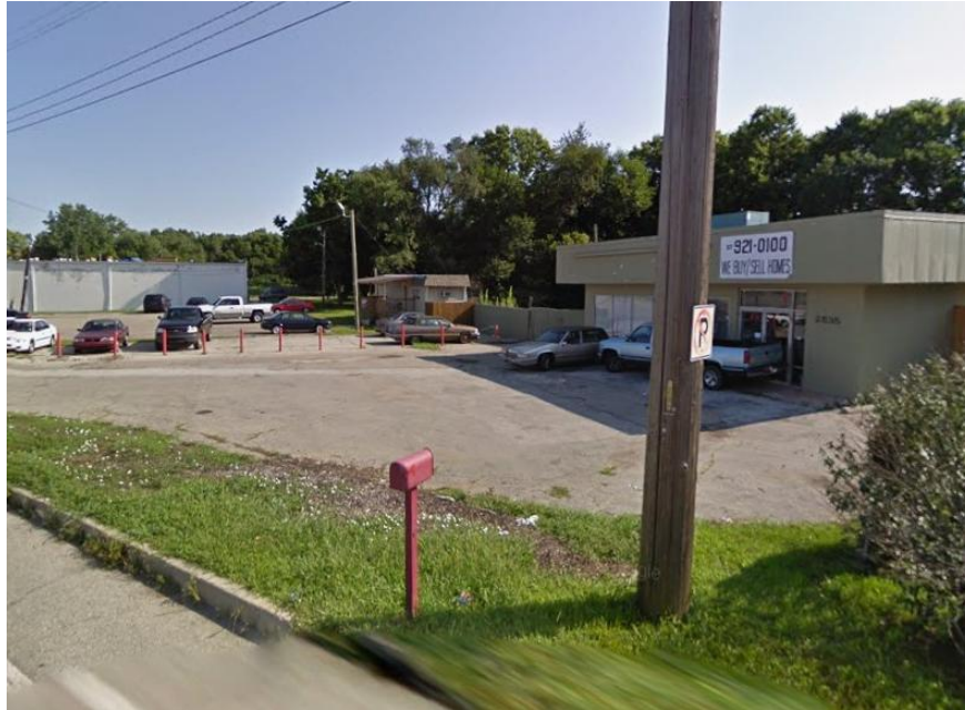
Photo 11: Adjacent Property to North (August 2009)
