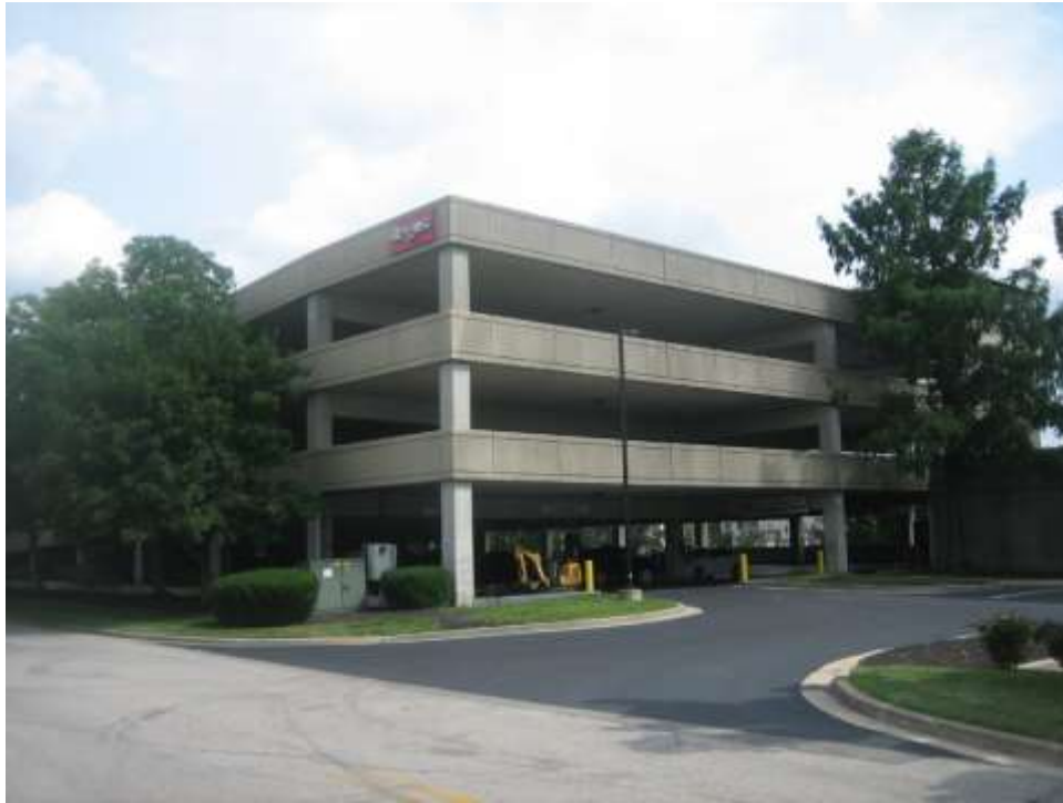
3815 River Crossign parkign garage north façade looking southeast
