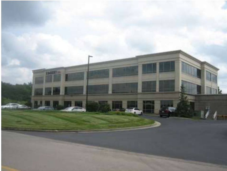
3925 River Crossing north façade, looking southeast
