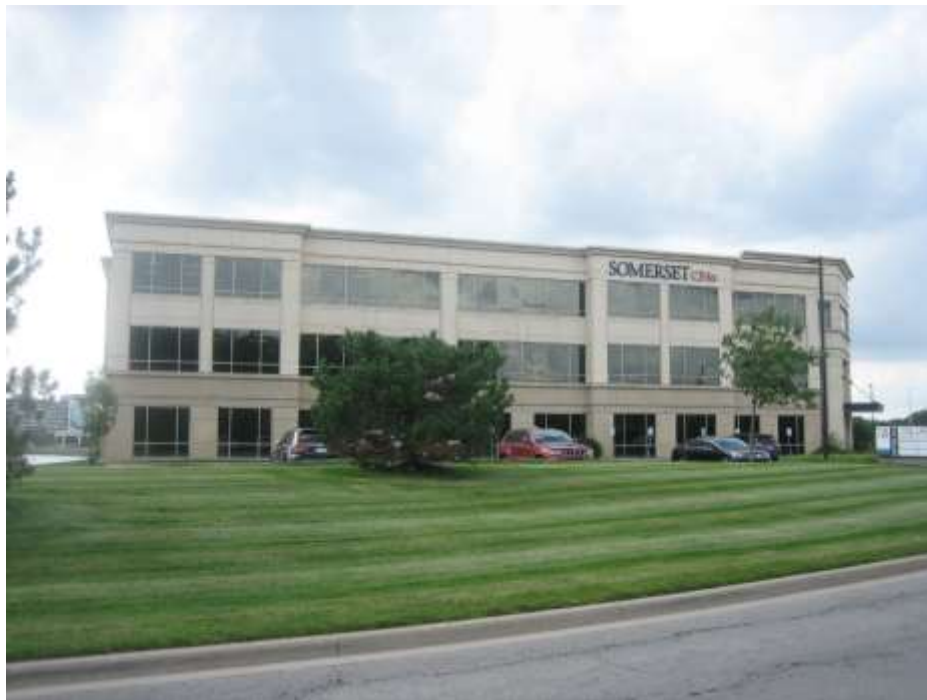
3925 River Crossing east façade, looking west
