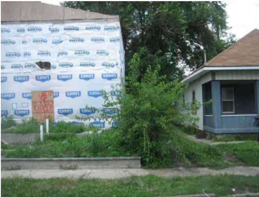
Subject property side setback, looking north.
