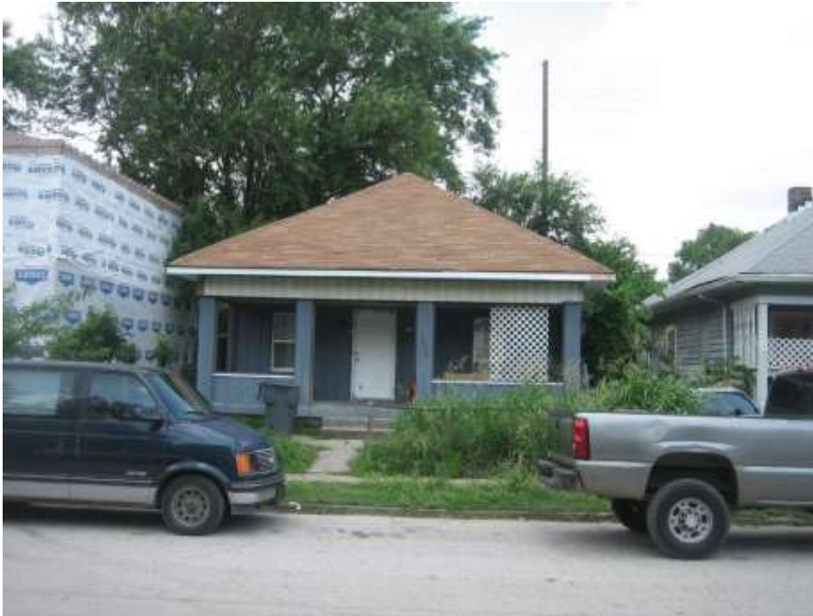
Adjacent property to the east, looking north.
