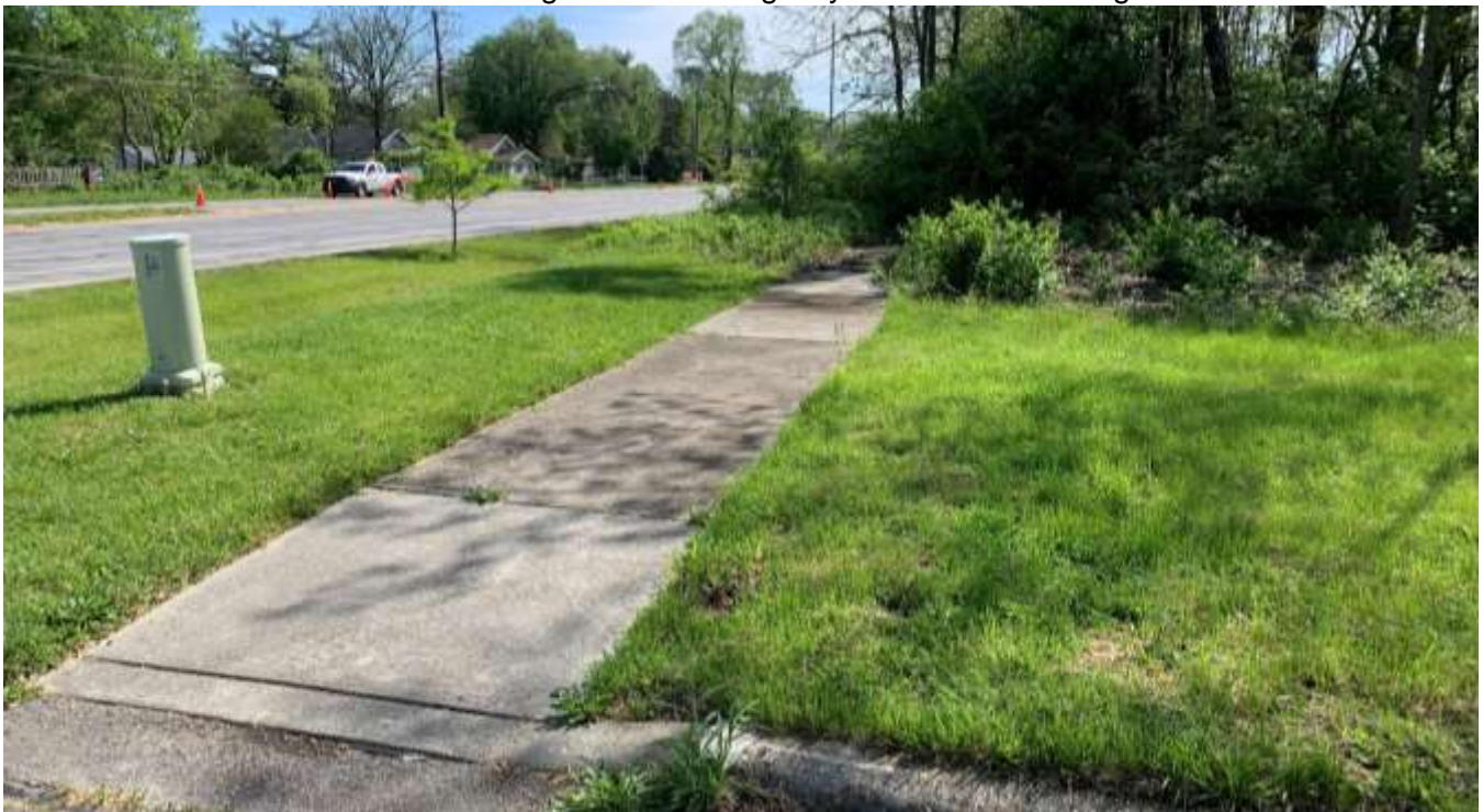
Photo of the existing sidewalk along Raymond Street looking east.
