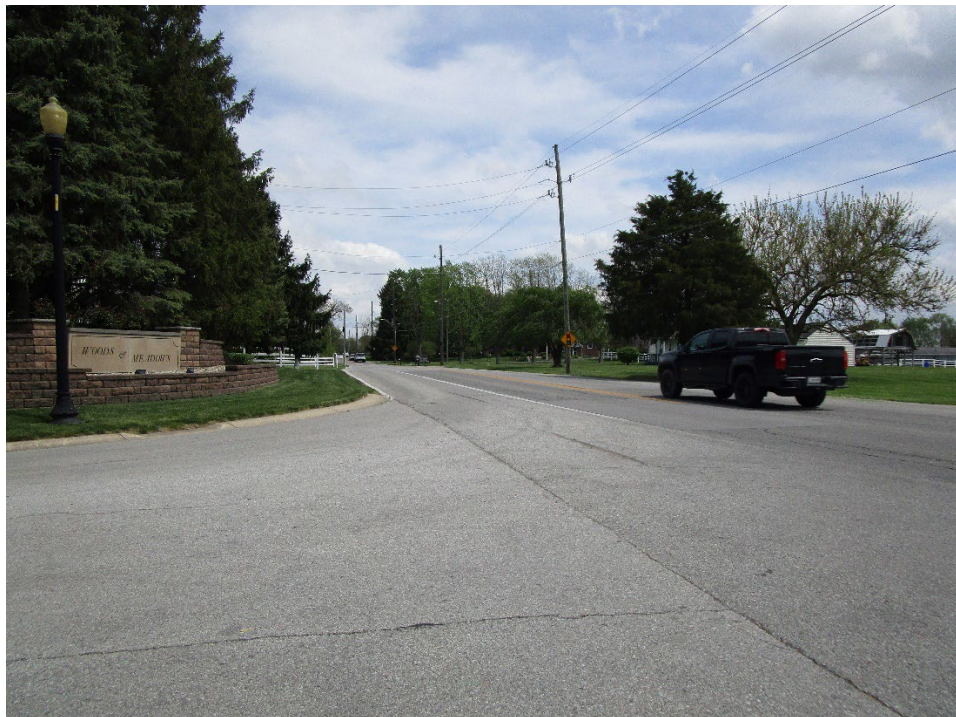
View looking east along East Edgewood Avenue
