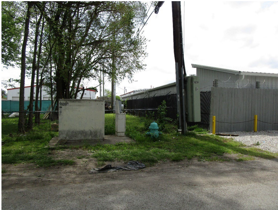
View of site looking south across West 17th Street
