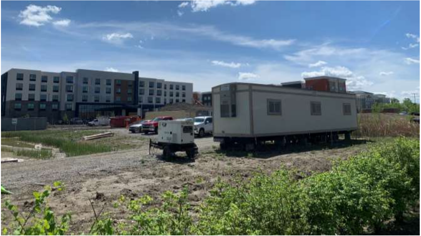
Photo of the subject site looking southeast.
