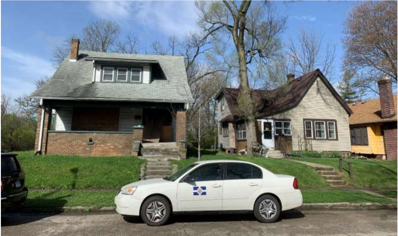
Photo of single-family dwellings west of the site
