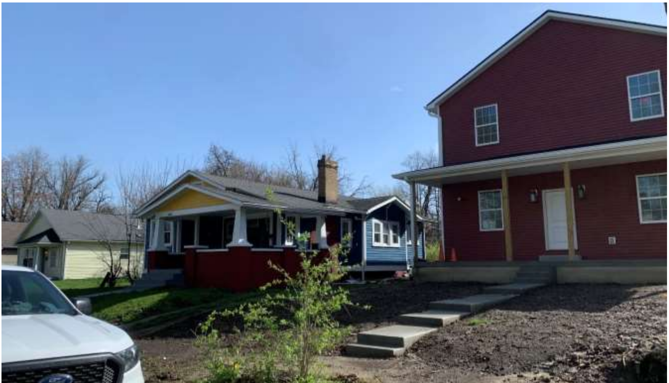
Photo of single-family dwellings north of 2255 North LaSalle Street.
