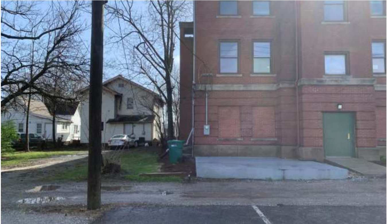
Photo of the rear building façade at 3350 Roosevelt Avenue.
