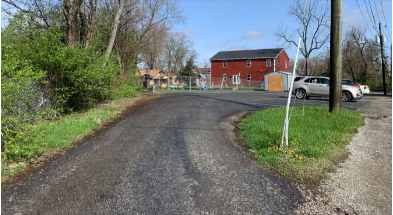
Photo of the parking lot at 3350 Roosevelt Avenue.
