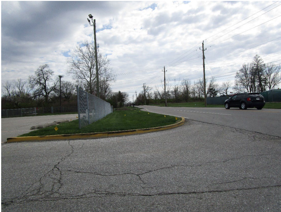
View looking south along South Franklin Road
