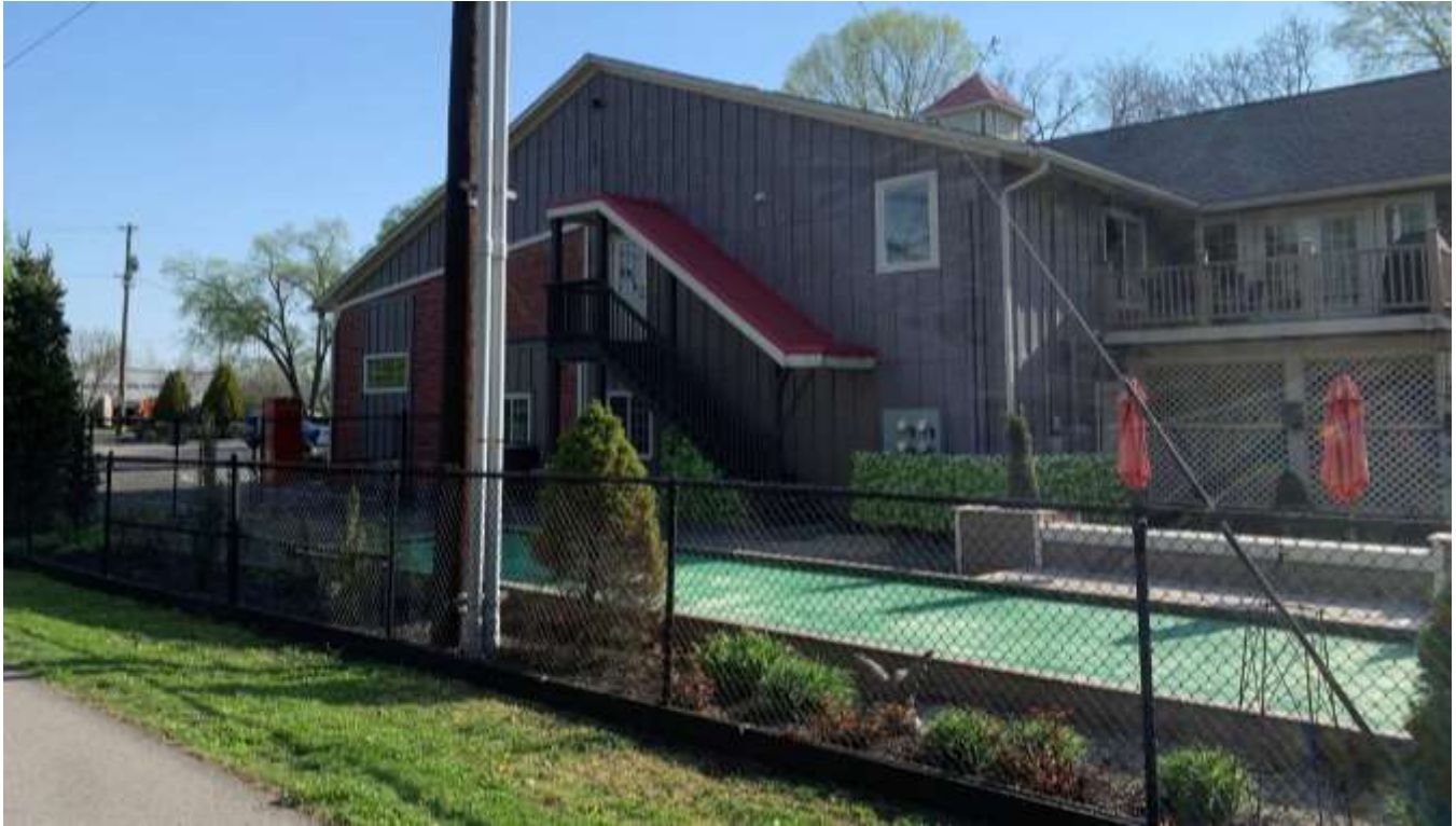
Photo of the west building façade and entrance to one of the units upstairs.
