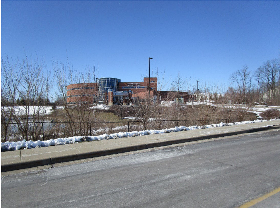
View of site looking northeast
