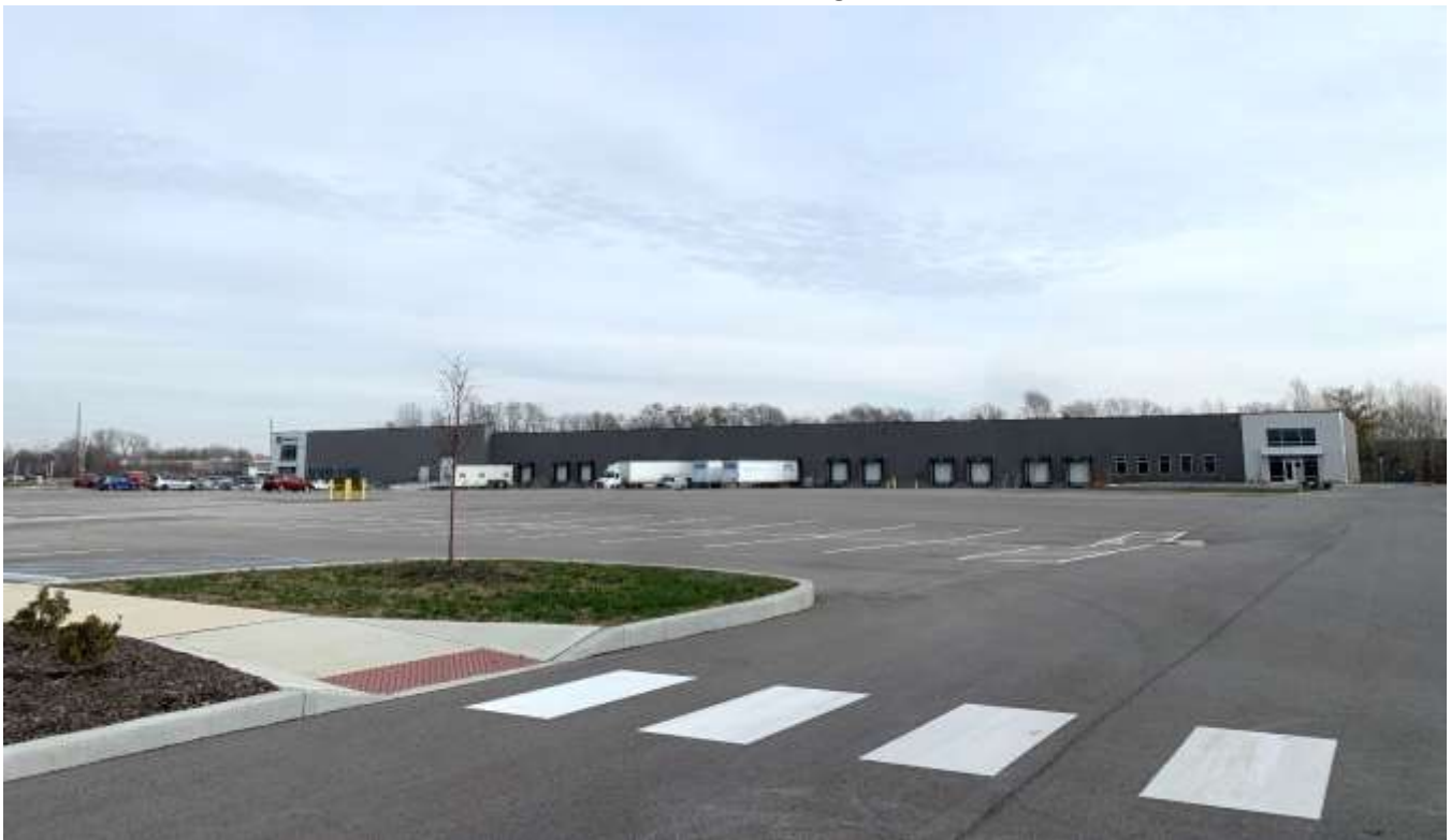
West building façade of Building 2 looking east.
