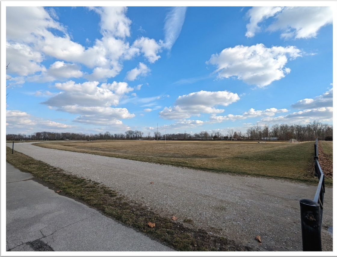
View of access road to be improved
