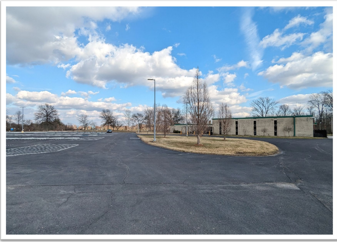
View from west entrance
