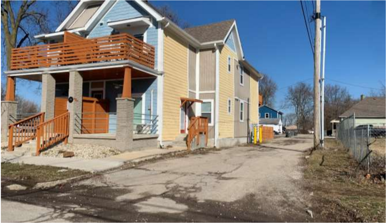
Photo of the dwellings west of the site across Bundy Place.
