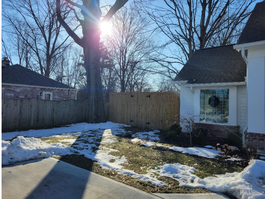
Photo 3: Fence at Southern Side Yard
