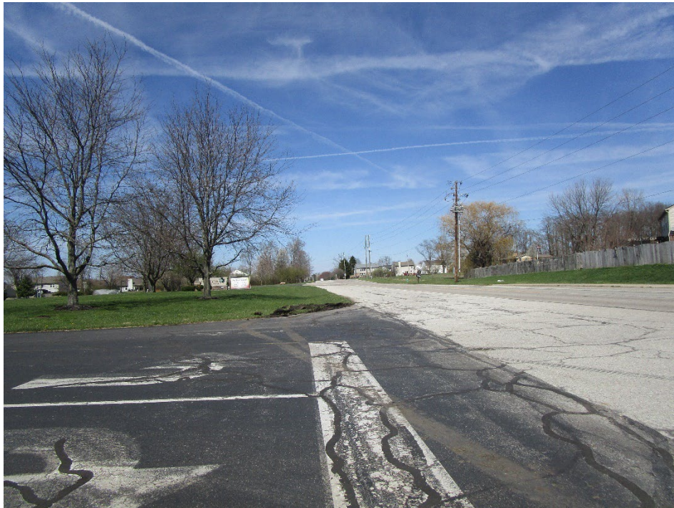
View looking north along Combs Road
