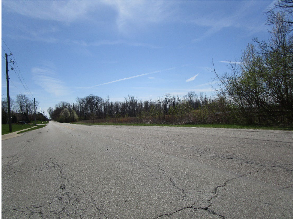
View of site looking southwest across Combs Road
