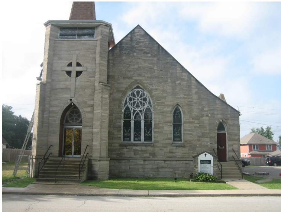
Photo of adjacent religious use to the west, looking south.
