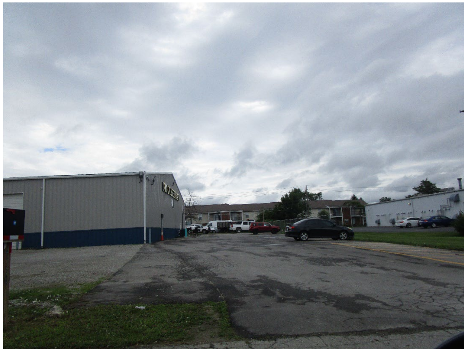
View looking north along eastern boundary
