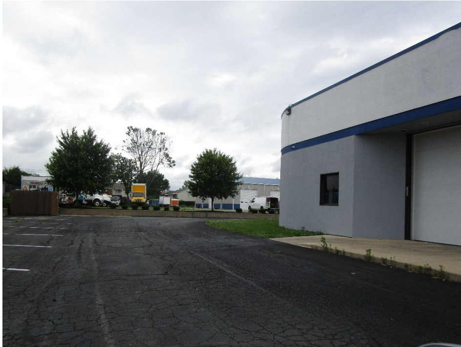
View of site (background) looking north from adjacent property to the south
