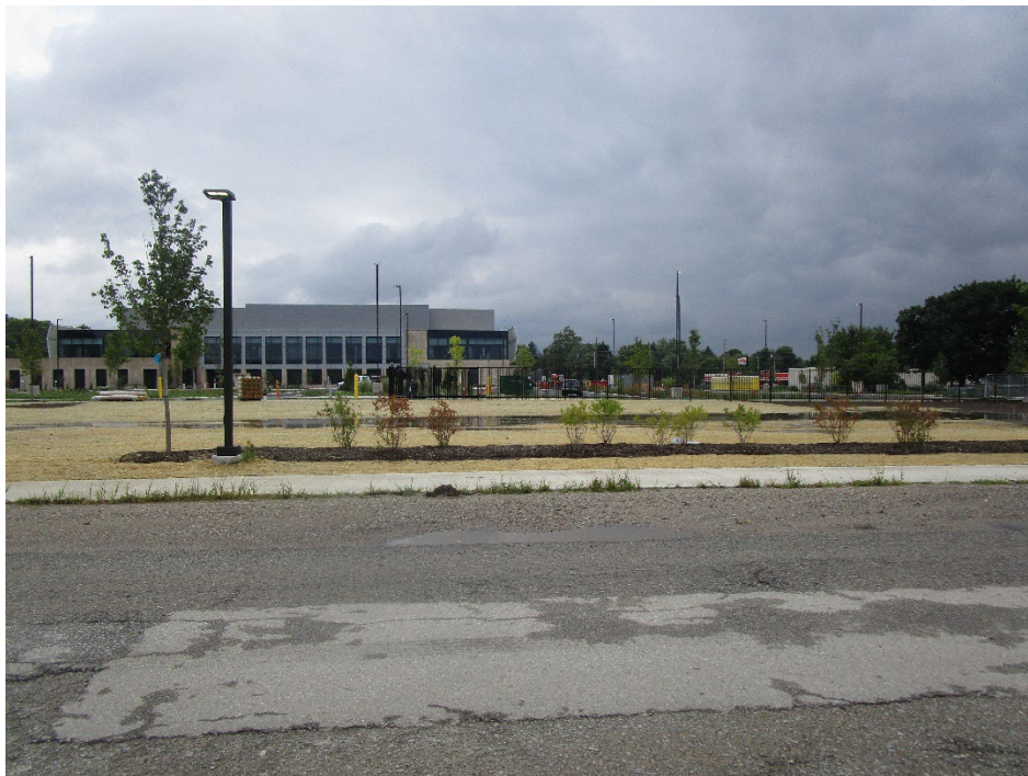
View of site looking south across East 39 th Street
