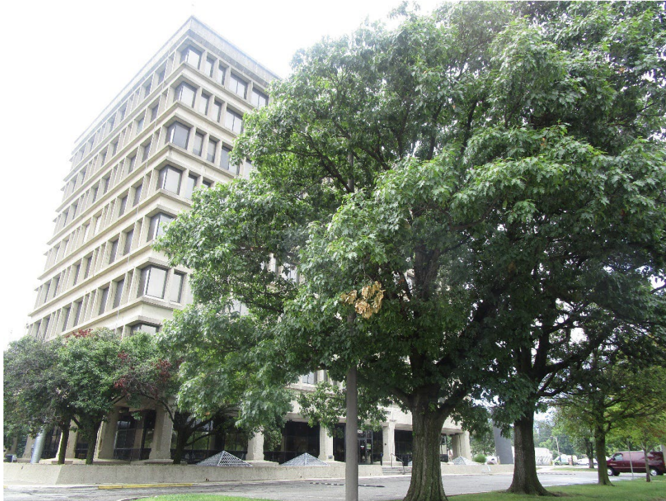
View looking northwest at the western building
