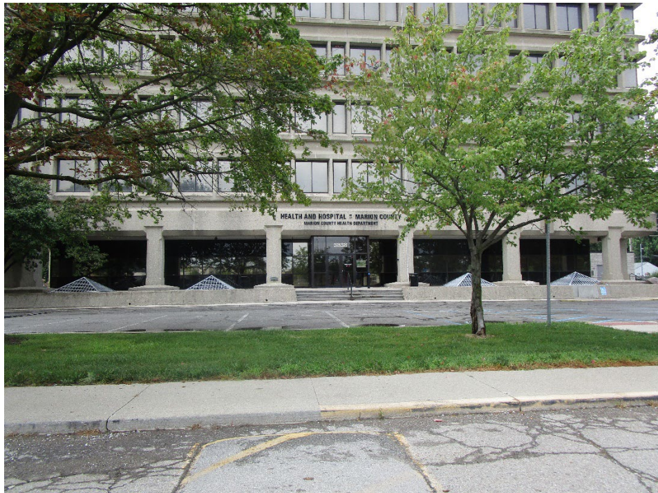
View looking west across North Rural Street of the western building
