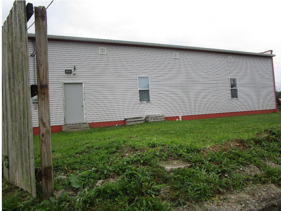
View of site looking southeast from north / south alley
