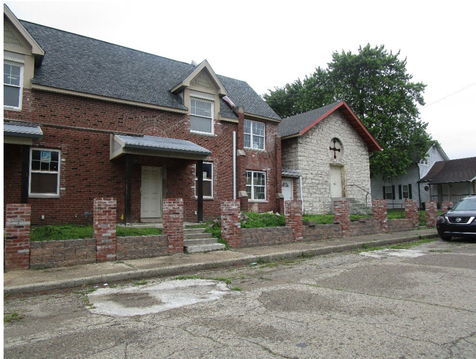
View of site looking northwest across Church Street
