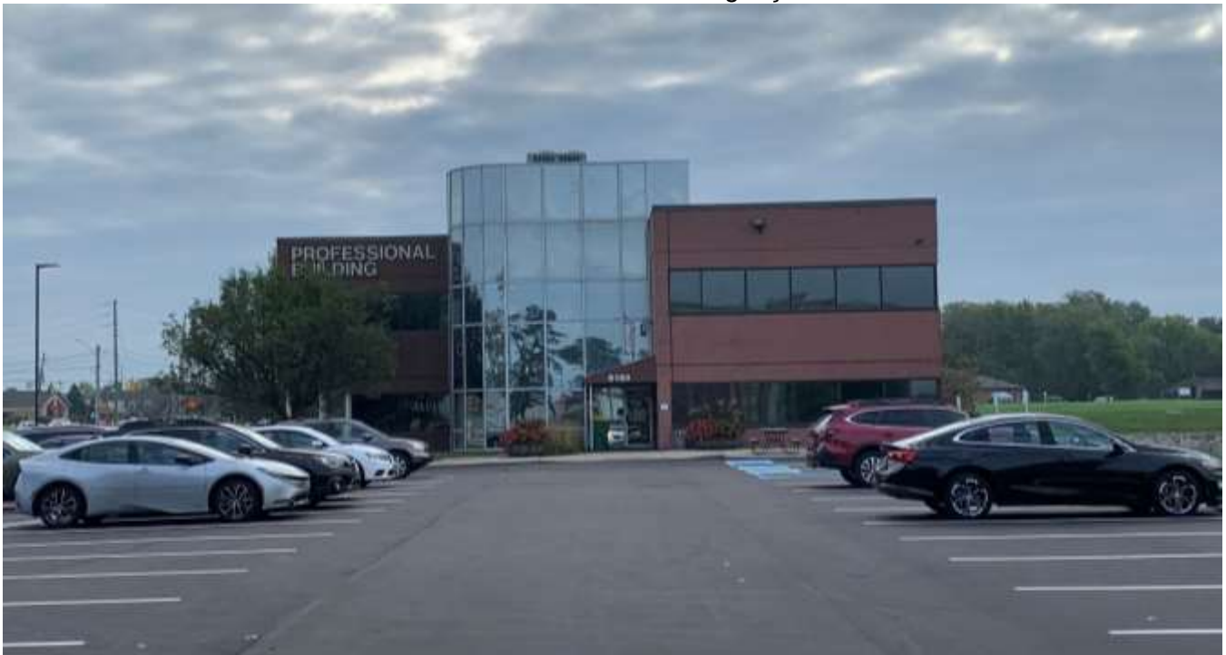
Photo of the western building façade.
