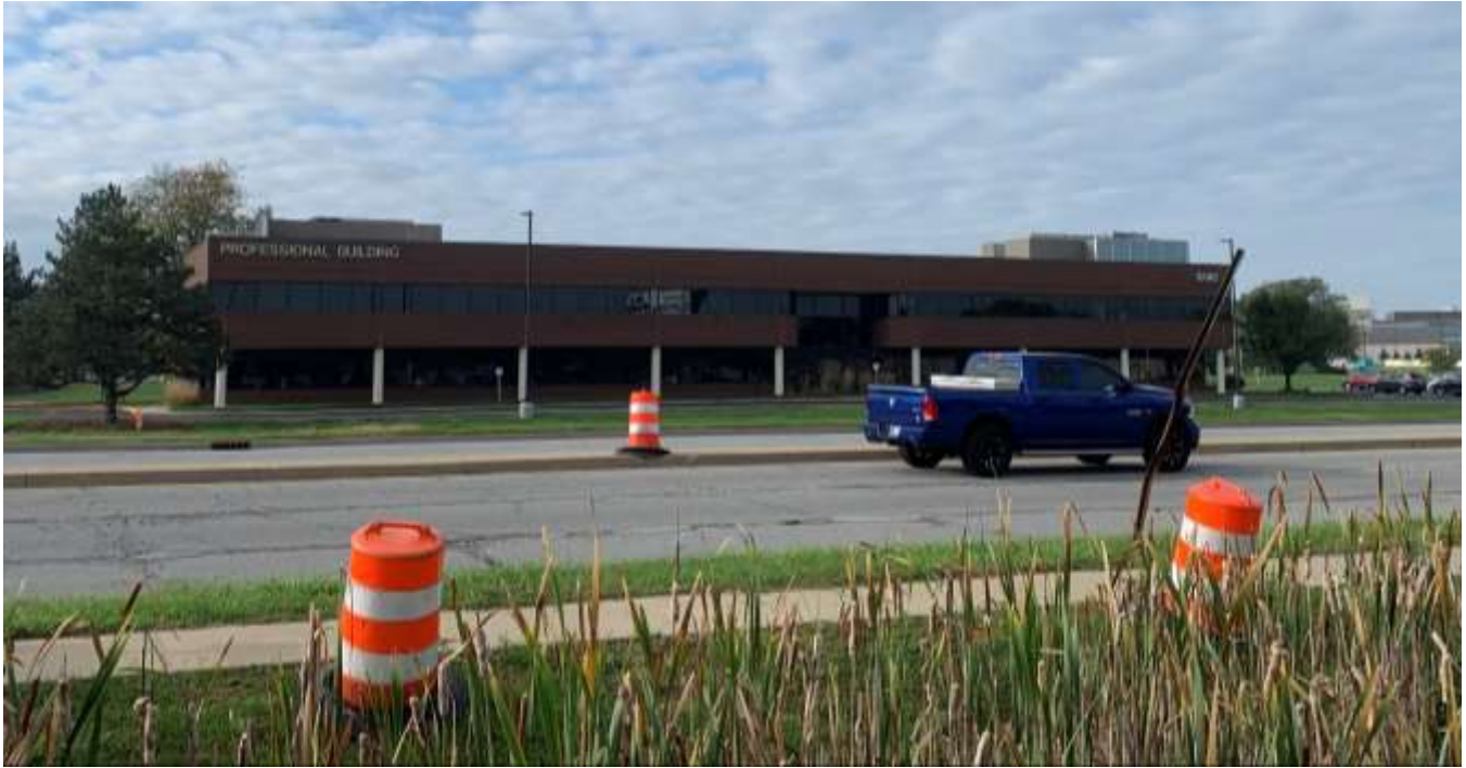
Photo of the northern building façade.
