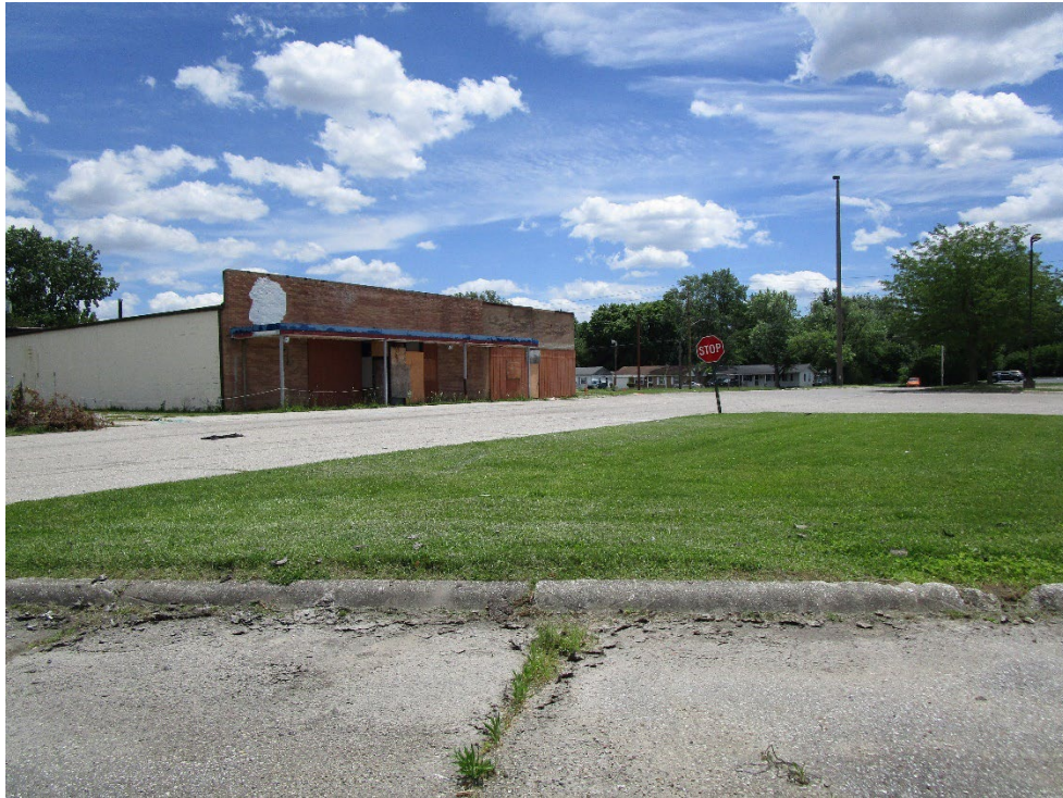
View of site looking southeast
