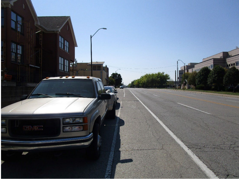
View looking south along South East Street
