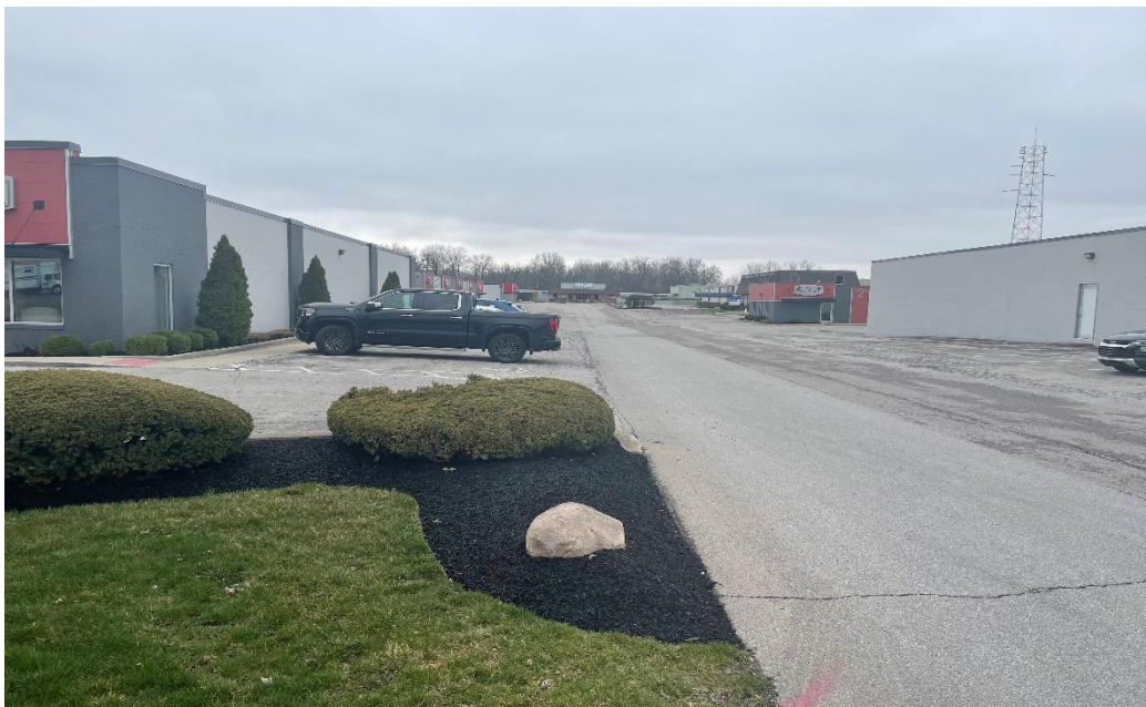
Photo Four: Example of Industrial Park Access Drive, Facing North
